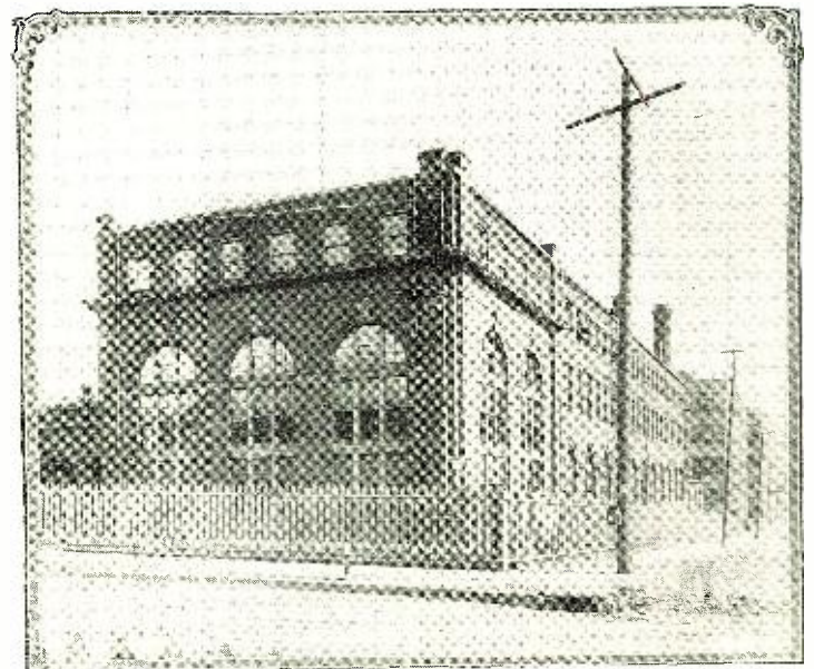
Exterior of the main building of the Edison laboratories at West Orange, N. J. Large as his laboratories are, Edison has yet succeeded in retaining individualistic inventive characteristics in his organization.
